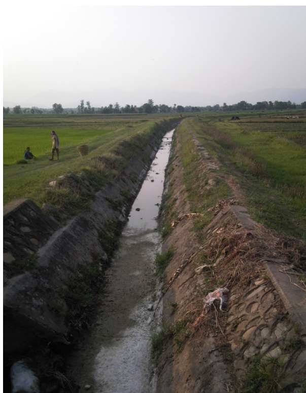
Picture 13: Concrete canal in PIS
