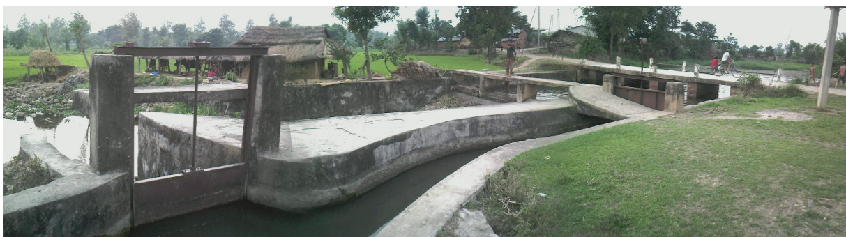
Figure 2.4: Intake structure (headwork) of Panchakanya Irrigation System
