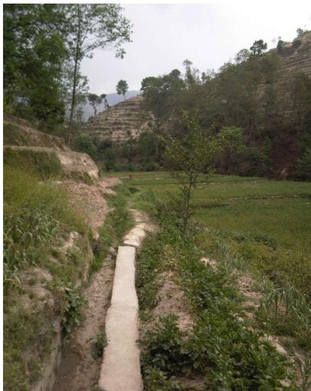
Picture 12: Partly constructed canal in TIS
