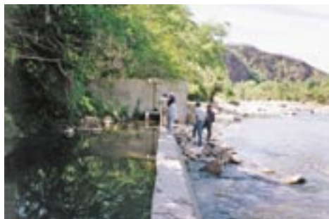
Photo 2.4 Intake in Naranjos Margen Izquierda irrigation system
