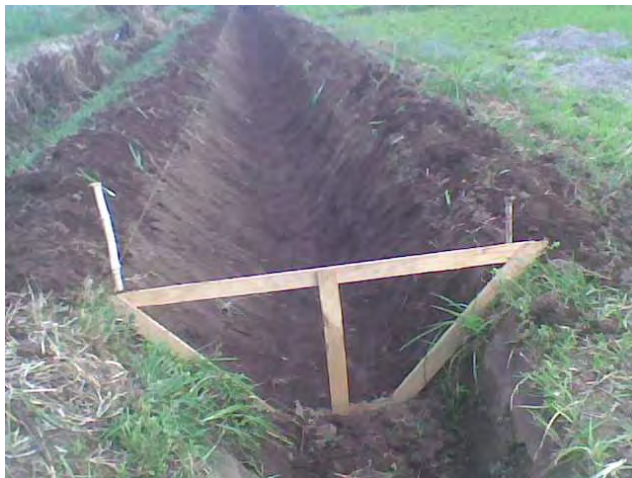
Photo 5.4: Wooden form used to set dimensions of canal
