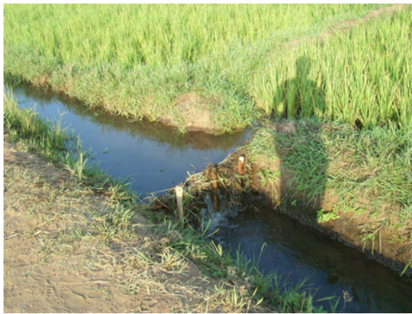
Photo 6.1: Structure in drain raising water into plot
