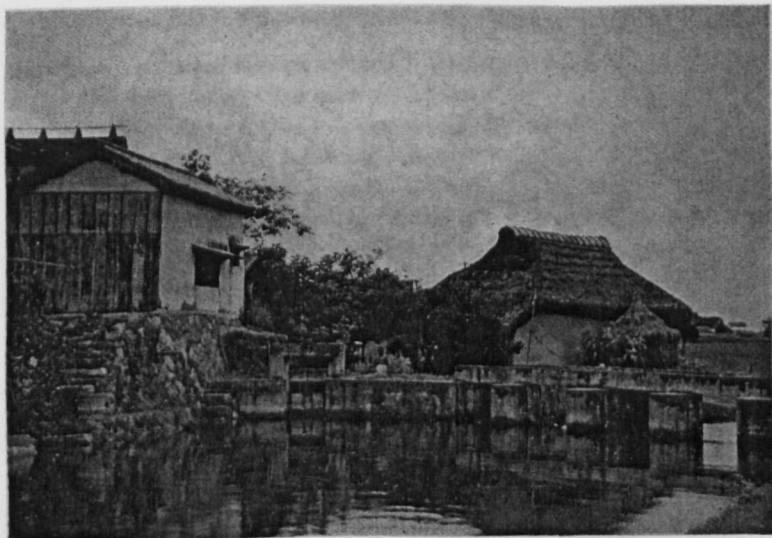
FIG. 10—Water divide at Mitsumizo. Steps and landing enable householders to use the backed-up water for laundry and other purposes.
