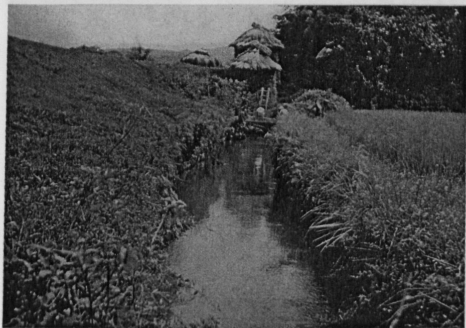
FIG. 9—Main canal passing under an elevated stream, the Chisui, in Oishi Village.
